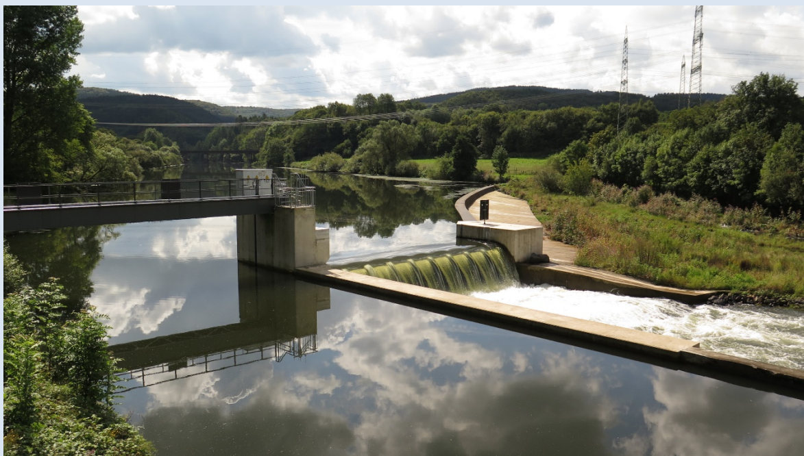
The headrace entrance, spillway gate and dam at the Unkelmühle power station in the Sieg. Photo by Eva B. Thorstad.
