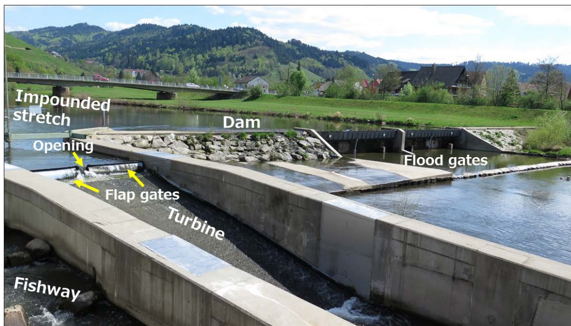
Figure 3.9. Photo of the dam and power station in Gengenbach, Kinzig, during low water discharge and the turbine in a lowered position. Photo: Eva B. Thorstad, taken 19 April 2015, at water discharge 17 \text{ m}^3\text{s}^{-1} .
