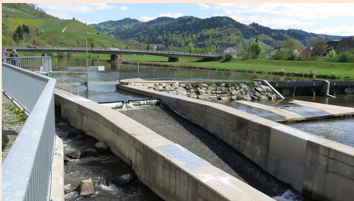
The fishway, section where the turbine is installed, dam and flood gates at Gengenbach power station in the Kinzig. Photo by Eva B. Thorstad.
